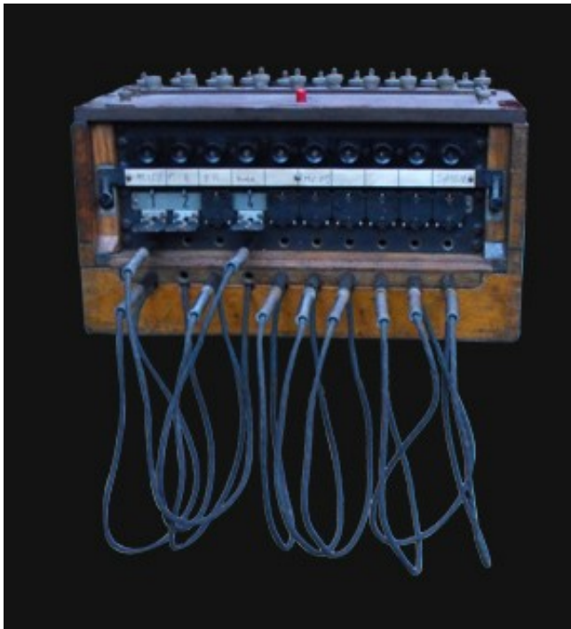
Ten-line Field Switchboard - Klappenschrank 33
