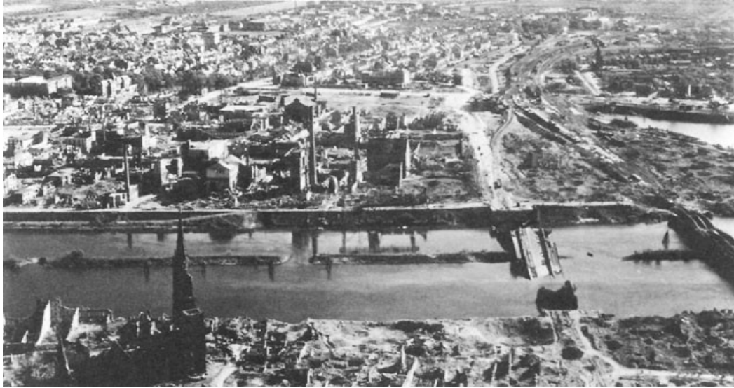
Ruined Bridges over the Weser River in Bremen
